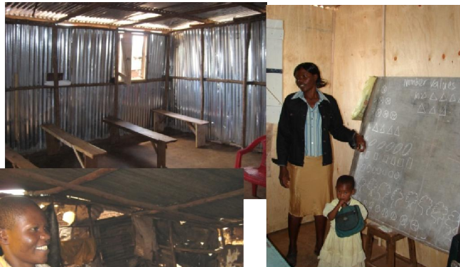
Inside the 10 x 14 feet KOPLWA centre in Kibera after the improvement of the infrastructure with concrete floor and more proper iron sheet walls and plywood interior.
