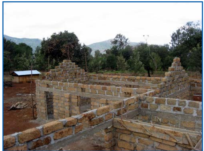
The first buildings of Ikumbo Secondary School under construction – July 2007
